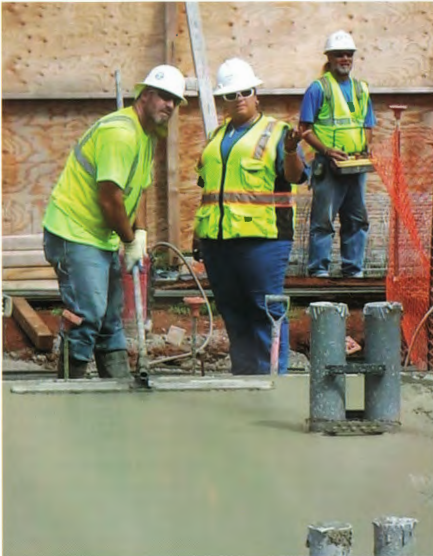
Nakeli Pascua coaches a worker on the Castner Substation project.
